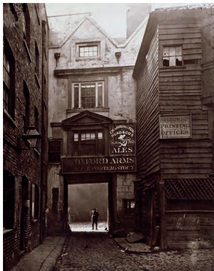
A. & J. Boal The Galleries of The Oxford Arms, Warwick Lane, looking from Warwick Lane c.1875 Carbon print
